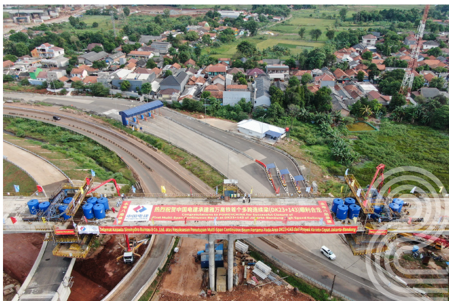
The multi-span rigid frame continuous beam for the No.2 Bridge of the Jakarta-Bandung High Speed Railway in Indonesia, on May 10, 2020
